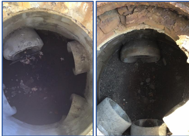
Figure 2-3 Example Manhole Condition
