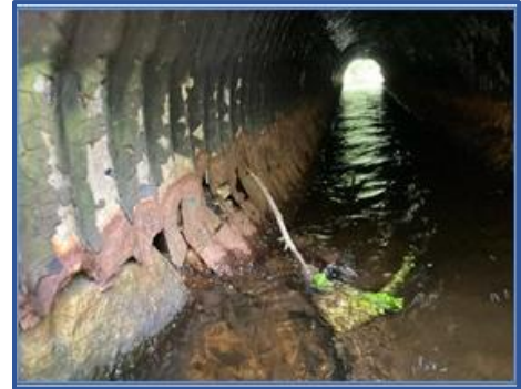
Figure 3-1 Example of invert deterioration in a CMP culvert (Culvert 66)
