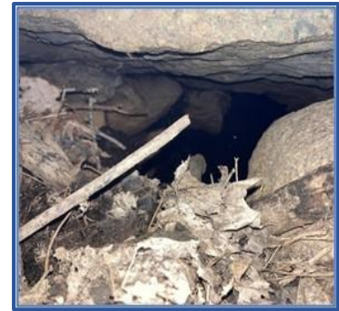
Figure 3-3 Example of Critical Obstruction at Culvert Inlet
