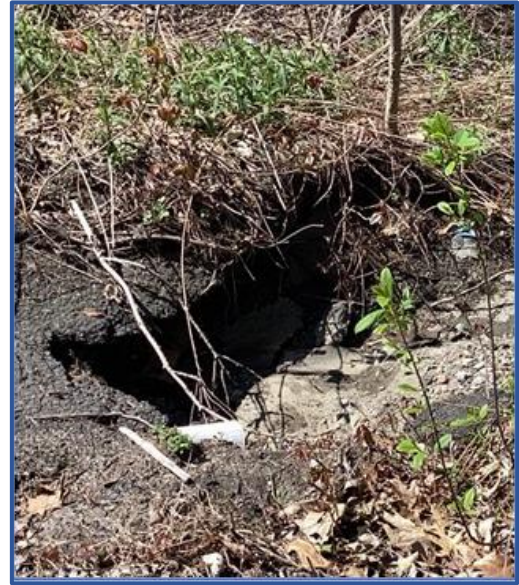
Figure 3-2 Example of a culvert with a tree at the headwall and critical roadway embankment (Culvert 4)
