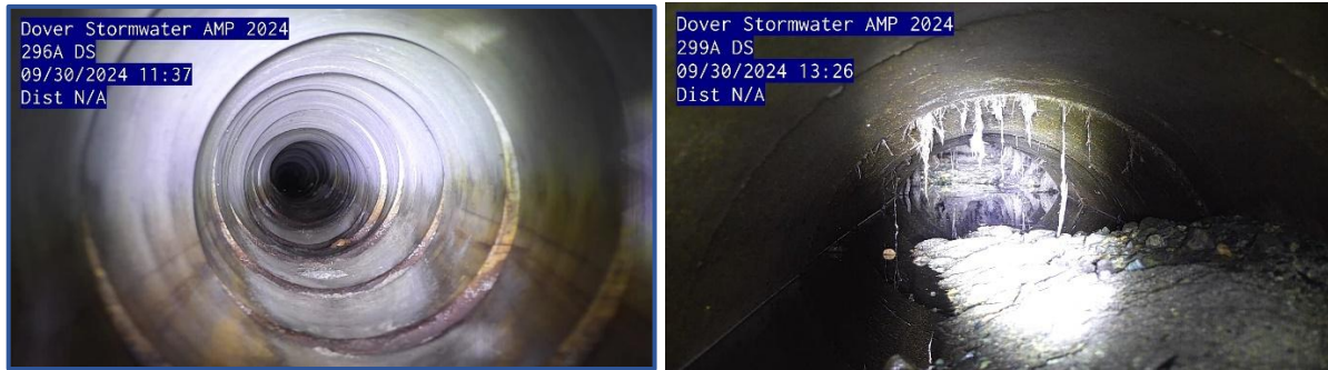
Figure 2-4 Example of Sedimentation in Pipes
